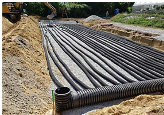
Manifolds being connected by flexible pipes.
