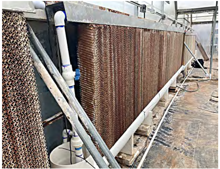
This evaporative greenhouse cooler's paper-like mat absorbs and evaporates water along one end wall of the greenhouse. Photo: Chris Lent, NCAT
