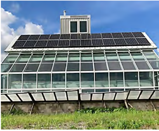
This passive solar greenhouse on Gib's Farm in Pennsylvania includes a thermal mass wall, steep-angle south-facing glazing, and a solar chimney for airflow and cooling in hot weather. Photo: Chris Lent, NCAT
